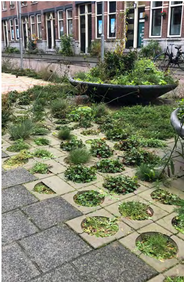
Figure 94. | Above and above right. Planting in footway spaces to encourage water infiltration - Rotterdam (paving specials www.struykverwoinfra.nl/ )
