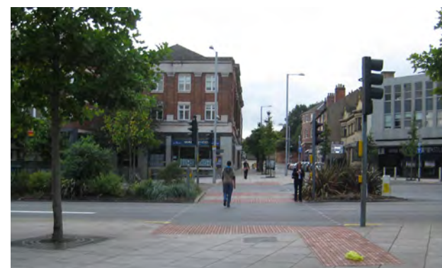
Figure 132. | Maid Marion Way, Nottingham, improvements: formerly a dual carriageway roundabout with underpasses for pedestrians, made into a surface signalised crossing without detriment to through traffic
