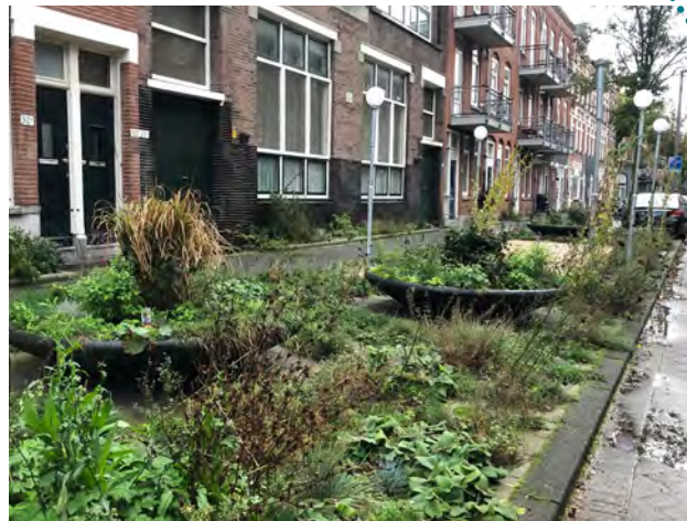
Figure 95. | example of a street sponge garden that threads small water attenuation features into narrow street spaces
